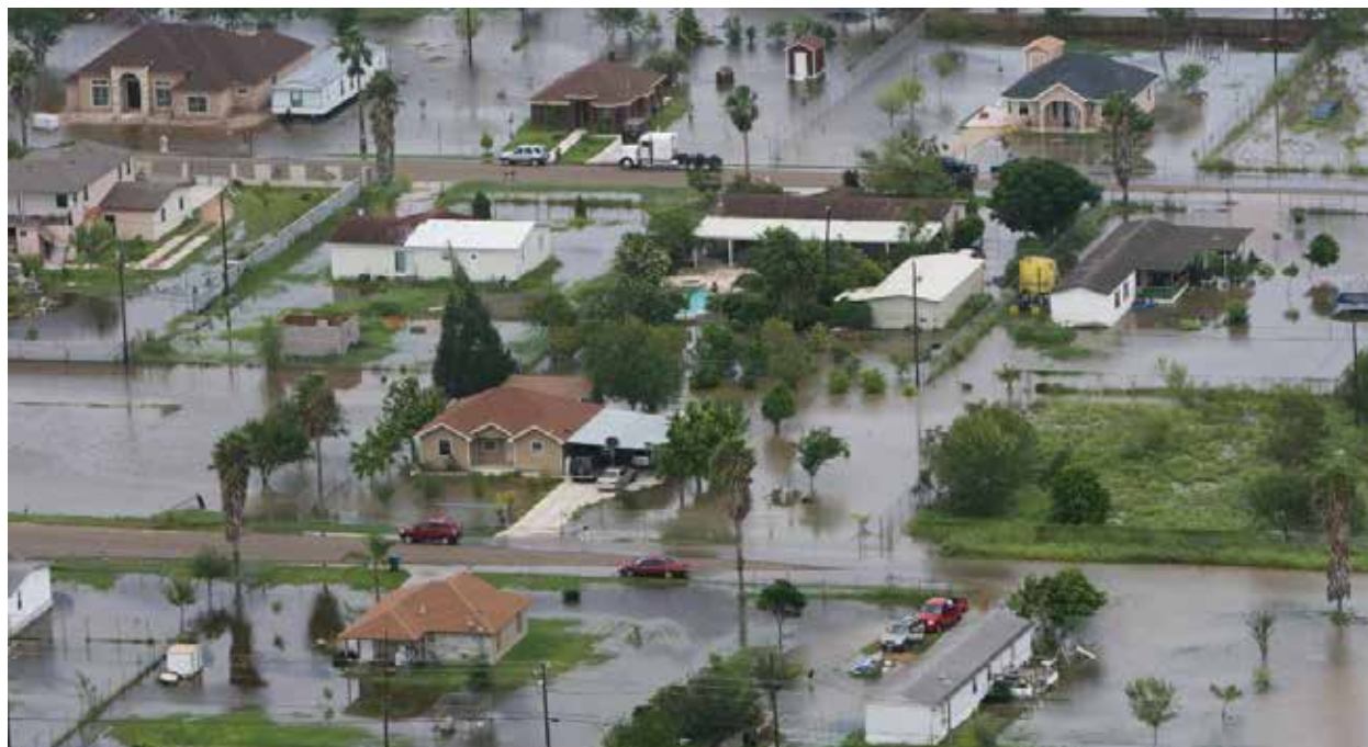
Flooding in Raymondville, another area of Texas prone to floods, during Hurricane Dolly (July 2008). The FEMA floodplain demarcates where development should occur, how high to build structures, and whether to buy flood insurance.
